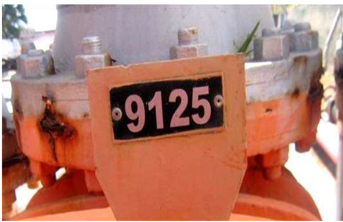
Pictures above show flange prepared for painting -notice the stripped surface
