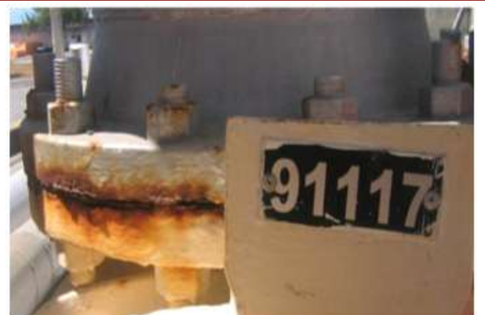
Pictured above are examples of anti corrosive gauze tape containing VCI foam (new and old)
