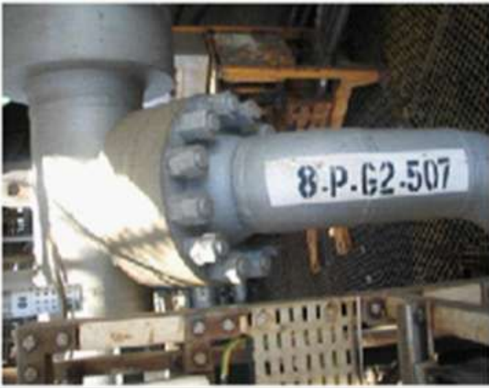
Pictured above are examples of anti corrosive gauze tape containing VCI foam (new and old)
