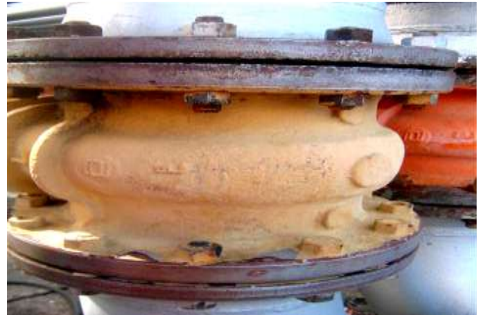
Pictures above show flange prepared for painting -notice the stripped surface
