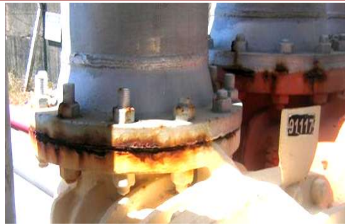
Flanges above are coated with anti-corrosion paint
